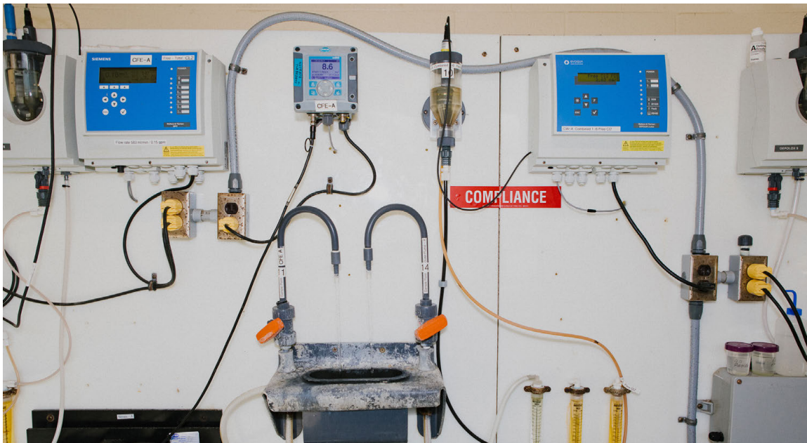
Left: Water analyzing equipment at the Chester Water Authority treatment plant. Right: Water being tested for chlorine residuals.
