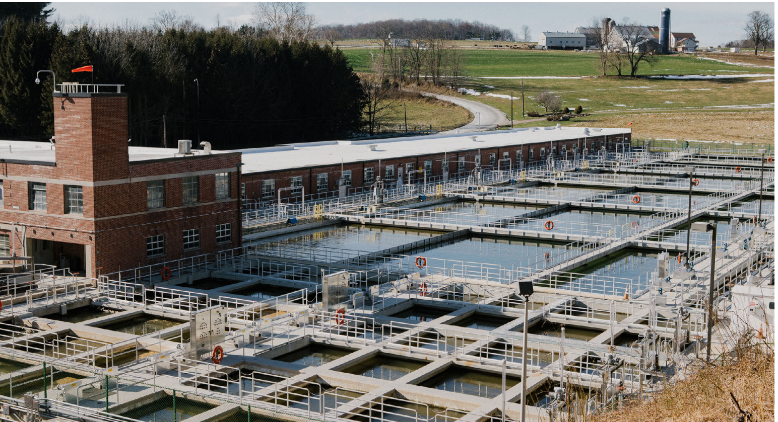
The outdoor conventional treatment pools at the Chester Water Authority (CWA) treatment plant in Nottingham, Pennsylvania.
