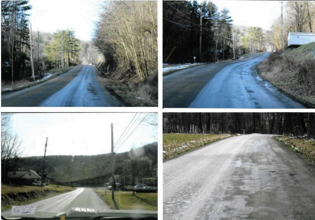
(March 2024 photos of road spreading)
